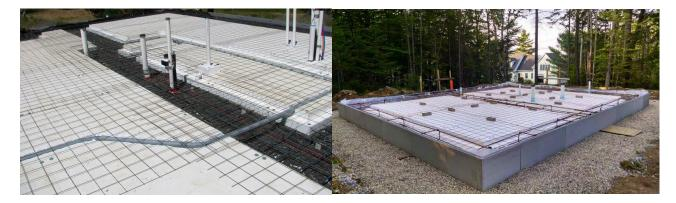
a layer of welded wire mesh over the entire extent of the slab. Anchor bolts for your exterior walls will be set into place now at the proper spacing. If you will have radiant heat in your slab then the network of heating tubing will also be installed at this stage.
