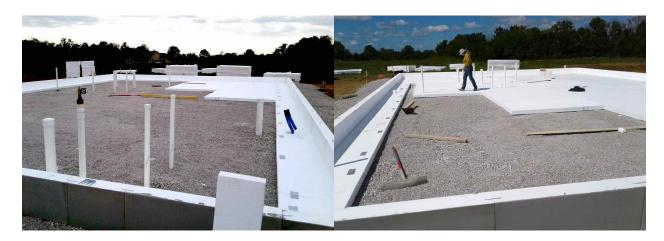
If you have any internal grade beams and column pads crossing the slab you must remember to use the high density Type IX foam under these foundation elements. You should have laid out these areas when you drew your layout diagram, so follow your drawing and put the high density foam in the proper locations.
